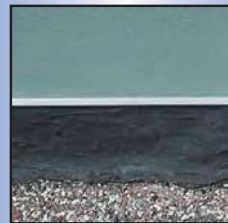
After - Repaired open joint in flashing by using the three-course flashing repair method.
