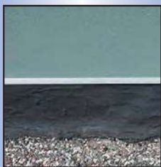
After – Installation of new Reinforced Perimeter Flashing Strip with butyl tape attached and EPDM flashing. New EPDM flashings are sealed to the underside of the existing EPDM field membrane.
