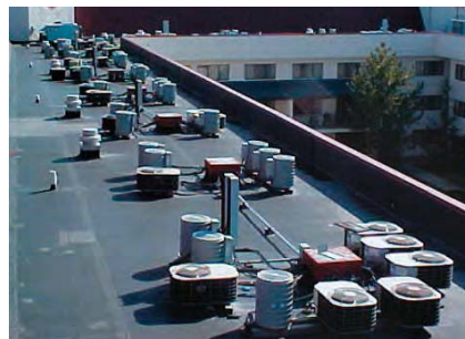
The huge amount of equipment placed on this EPDM roof will require careful monitoring by maintenance personnel.
