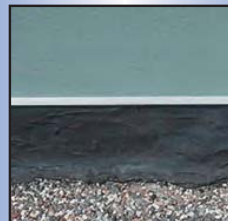
After - Repaired open joint in flashing by using the three-course flashing repair method.
