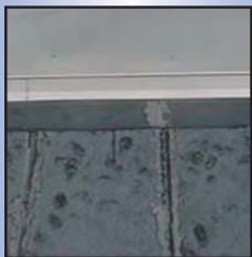
Before - Open seams and deteriorated surface on modified bitumen membrane on sloped wall
